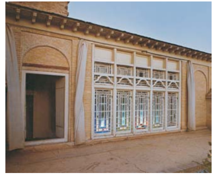
The upper portion of the building where the Báb declared His mission on 23 May 1844 in Shiraz, Iran, before its destruction in 1979
